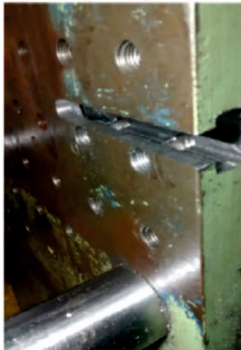
5. Cutting of 'T-slot' completed
